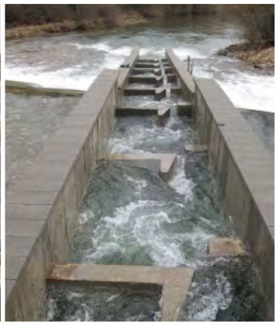
Figure 8. Pool and weir fish ladders: “submerged spillway and bottom orifice” in the River Duero (Guma, Burgos) and “vertical slots” in the River Porma (Vegas del Condado, Leon)
