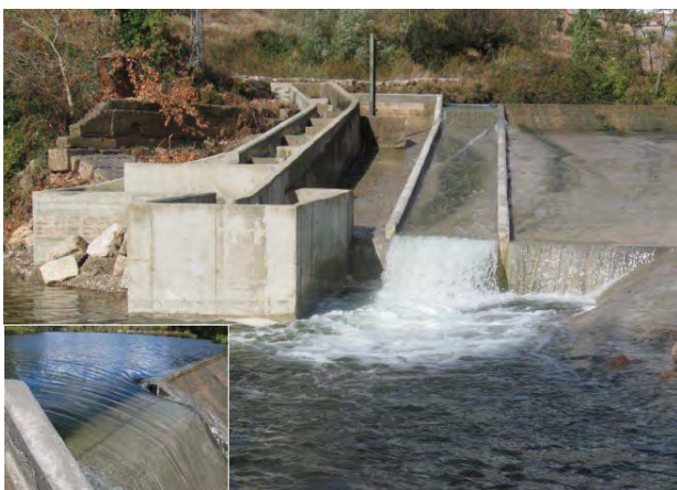
Figure 11. Fish slide for downstream movements in Torquemada (River Pisuerga, Palencia). It is positioned near the turbine outlet and it is occasionally used to add greater volume to the fish ladder entrance, increasing the “attraction”.
