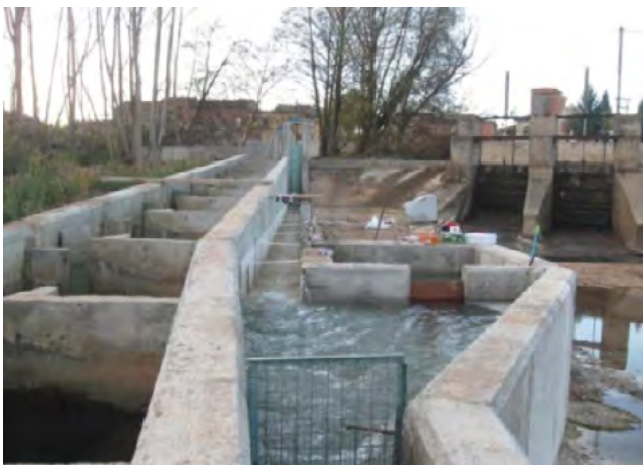
Figure 15. Fish swimming flume in Vadocondes (River Duero, Burgos), the first voluntary swimming channel in Europe. The swimming capacity at different flow speeds is analysed from the information collected by a PIT tag system and video cameras (see the next page).
