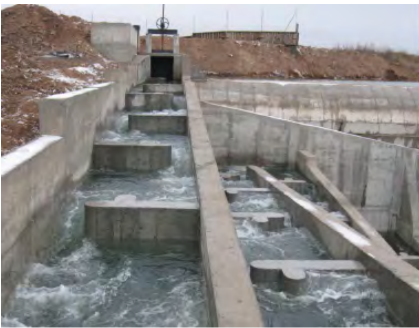
Figure 8. Pool and weir fish ladders: “submerged spillway and bottom orifice” in the River Duero (Guma, Burgos) and “vertical slots” in the River Porma (Vegas del Condado, Leon)
