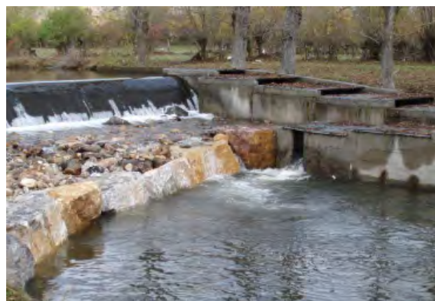
Figure 3. Example of two correctly located fish ladders in Peñafiel (river Duero) and in Puebla de Lillo (river Porma). Wherever possible, the fish pass entrance should be placed next to the riverbank and near the face of the dam, making it easy to locate for the fish.
