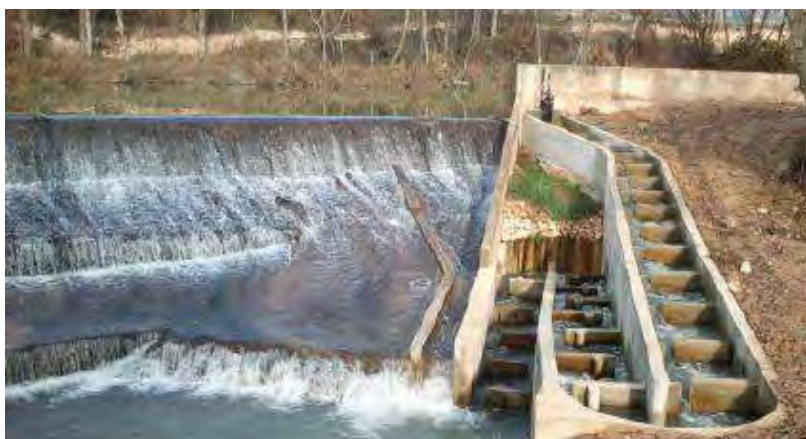
Figure 3. Example of two correctly located fish ladders in Peñafiel (river Duero) and in Puebla de Lillo (river Porma). Wherever possible, the fish pass entrance should be placed next to the riverbank and near the face of the dam, making it easy to locate for the fish.
