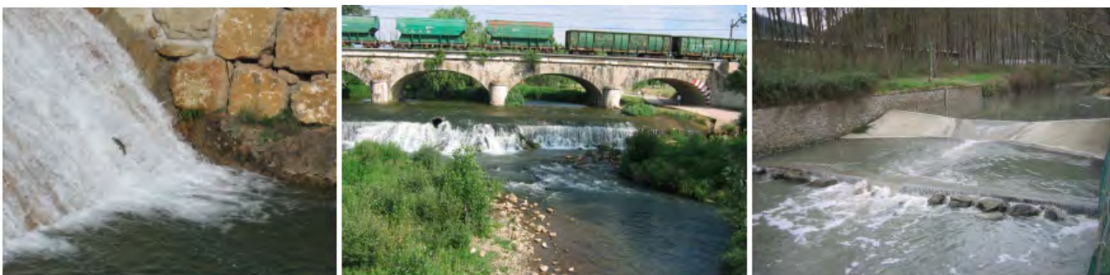
Figure 1. Main obstacles that limit the movement of the fish: dams, irrigation dams, bridge foundations,
