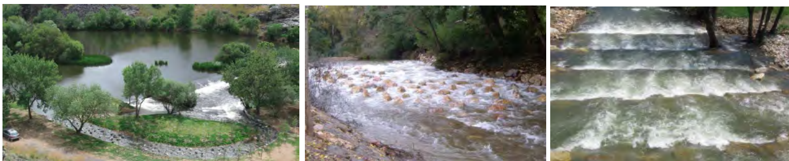
Figure 6. An example of nature like fish passes: artificial river in the River Tormes in El Marín (left); stone ramp in the River Najerilla in Torremontalbo (centre) and pre-dams in the River Pisuerga in San Salvador de Cantamuda (right)
