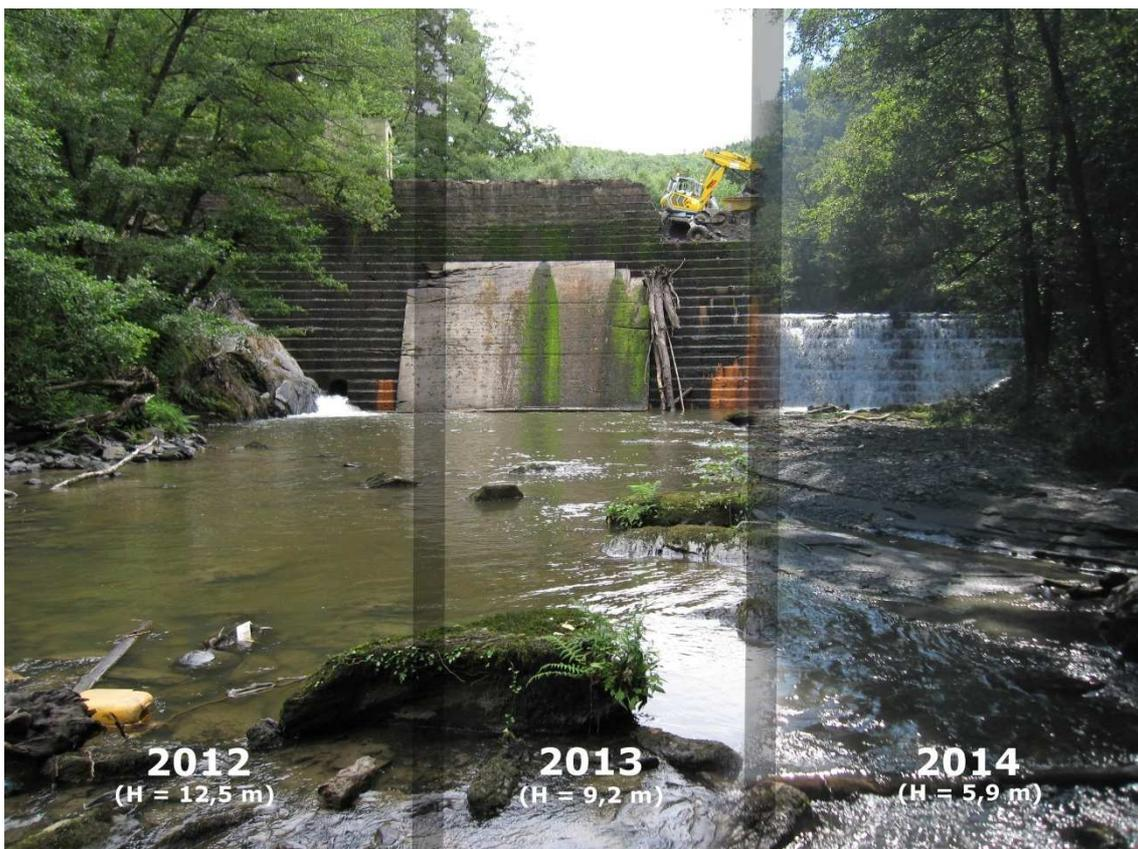
Figure 30. stages of the Inturia dam Removal. The image shows the comparison with the initial state and the results of the first two stages of the project and also the reduced height in each year. Photo credits: Irekia.
