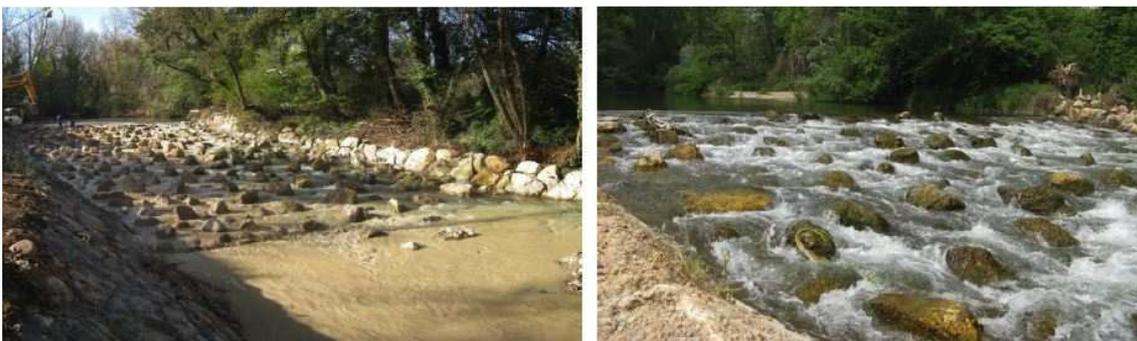
Figure 37. Rock ramp in the Najerilla River with a low flow (left) and with a higher flow (right).
