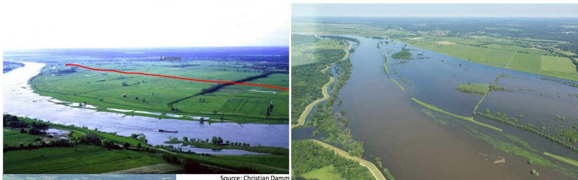
Figure 1. The area affected by the levee set-back: on the left, before the works; on the right, the openings shown at work during a flood. The red line on the left picture indicates the position of the new levee (sources, left: Christian Damm; right: Nora Künkler).
