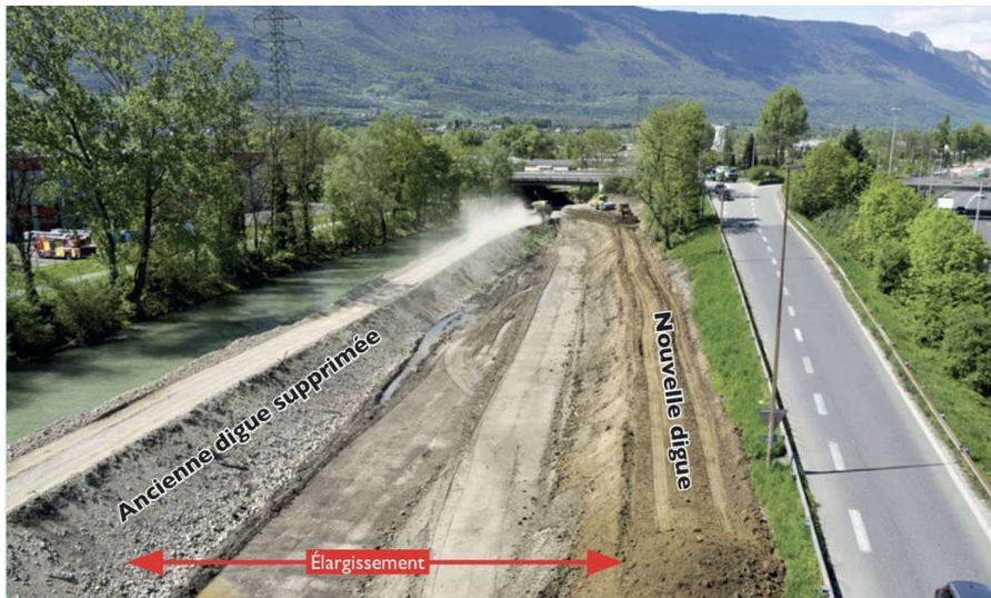
Figure 5. Construction works: setting back the levee.
