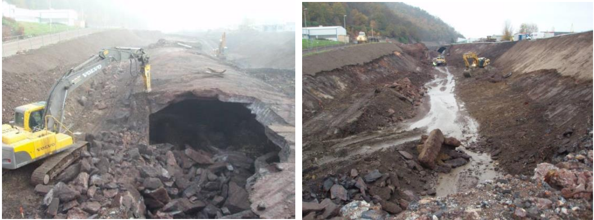
Figure 22 The reopening works at the Ondaine river
