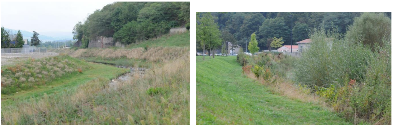
Figure 23 The restored stretch just upstream the deculverted section
