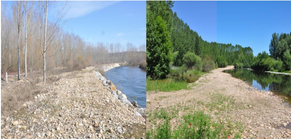
Figure 4. River bank protections were also removed along the river: on the left, the situation before the project; on the right, the river is reconnected to its floodplain (source: Duero River Basin Authority – Confederación Hidrográfica del Duero, CHD).
