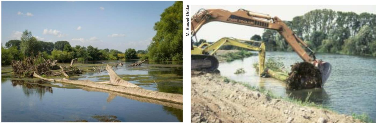
Figure 16. Large Woody Debris were put in place to initiate natural dynamics (source, M. Bunzel-Drüke).
