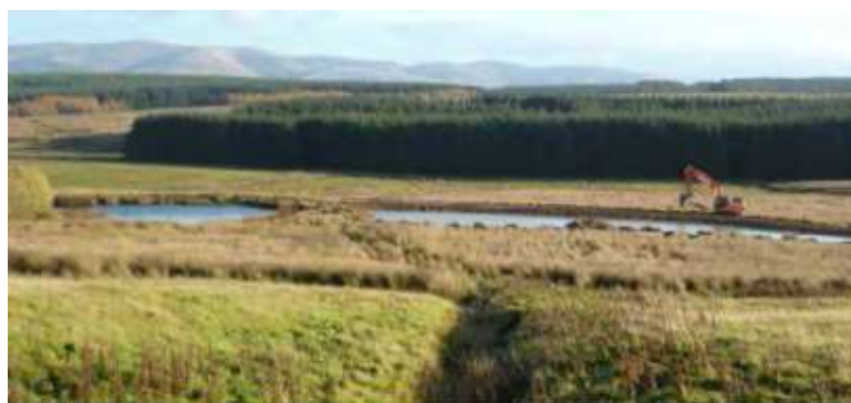
Figure 11. Construction of new ponds in the upper catchment (source: Eddleston Water Interreg Project Report 2016).
