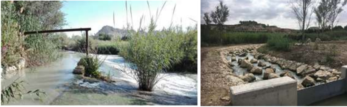
Figure 9. Azud Archena weir, on the left, and lateral fish bypass for Archena weir, on the right (source: Segura River Basin Authority – Confederación Hidrográfica del Segura).
