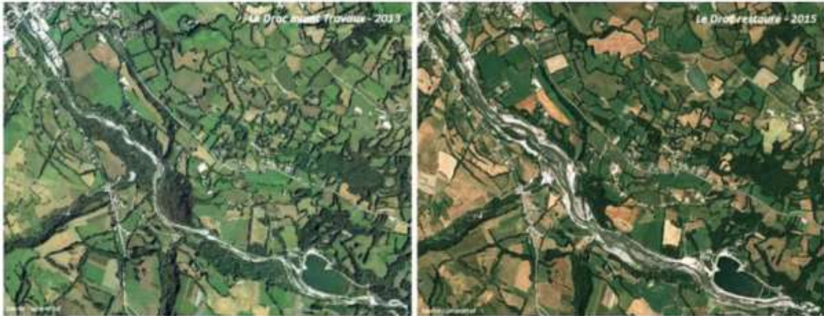
Figure 4. On the left panel, aerial view on the single channel Drac prior the 2013 intervention; the Champsaur dam can be recognized in the bottom right corner. The river flows towards the top of the picture. On the right panel, the same reach after the intervention (source: French geoportal).
