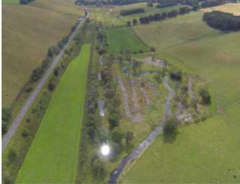
Figure 12. Re-meandered section of Lake Wood, with the old channel on the left (source: Eddleston Water Interreg Project Report 2016).
