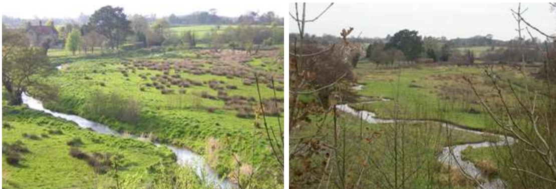
Figure 13. Re-meandered reach of the River Glaven at Hunworth: (a) In January 2009, prior to the rehabilitation project, on the left, and in December 2010, after re-creation of meanders in August on the right (source: modified by Champkin et al., 2018).
