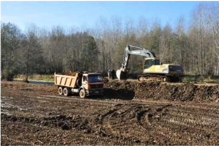
Figure 7. An artificial levee is lowered to recover lateral connectivity (source: Duero River Basin Authority – Confederación Hidrográfica del Duero).
