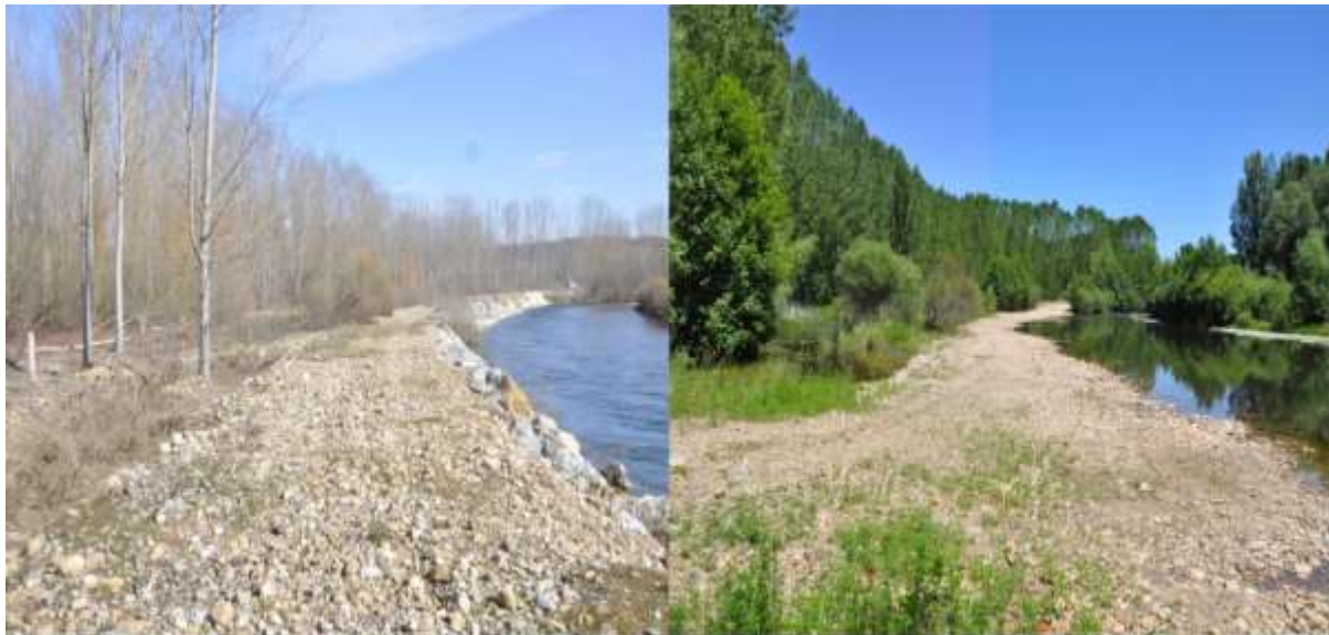
Figure 8. River bank protections were also removed along the river: on the left, the situation before the project; on the right, the river is reconnected to its floodplain (source: Duero River Basin Authority – Confederación Hidrográfica del Duero).
