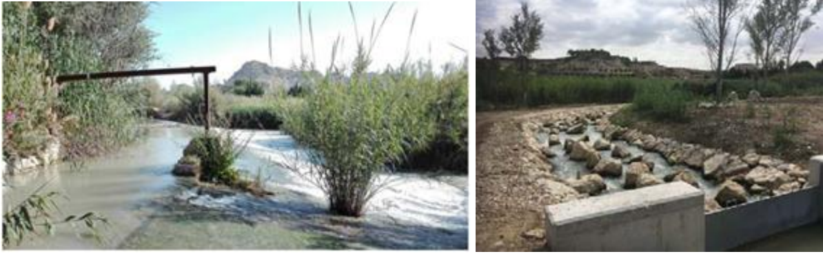
Figure 9. Azud Archena weir, on the left, and lateral fish bypass for Archena weir, on the right (source: Segura River Basin Authority – Confederación Hidrográfica del Segura).
