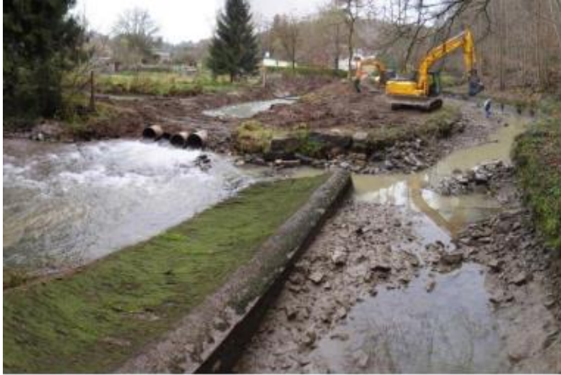
Figure 1. Works for weir removal at Spontin (source: LIFE project «Walphy» Layman's report).
