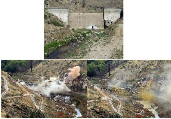
Figure 32. Moment of the demolition of Robledo de Chavela dam. The first photo shows the dam before its removal. The second picture shows the demolition moment and the third the state of the dam after demolition. Photo Credits: Ministry of Agriculture and Fishing, Food and Environment (MAPAMA).
