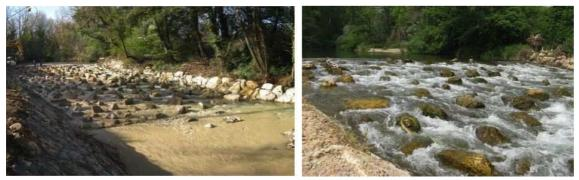
Figure 37. Rock ramp in the Najerilla River with a low flow (left) and with a higher flow (right). Photo credits: Pedro Boné.
