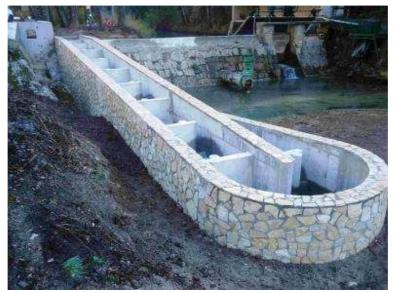
Figure 39. The fishpass built in Las Librerías weir on the Guadiela River. Photo credits: Europa press/JCCM.
