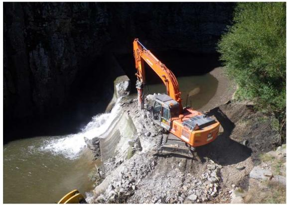
Figure 34. Image of the removal works of La Gotera dam. Photo Credits: Ministry of Agriculture and Fishing, Food and Environment (MAPAMA).
