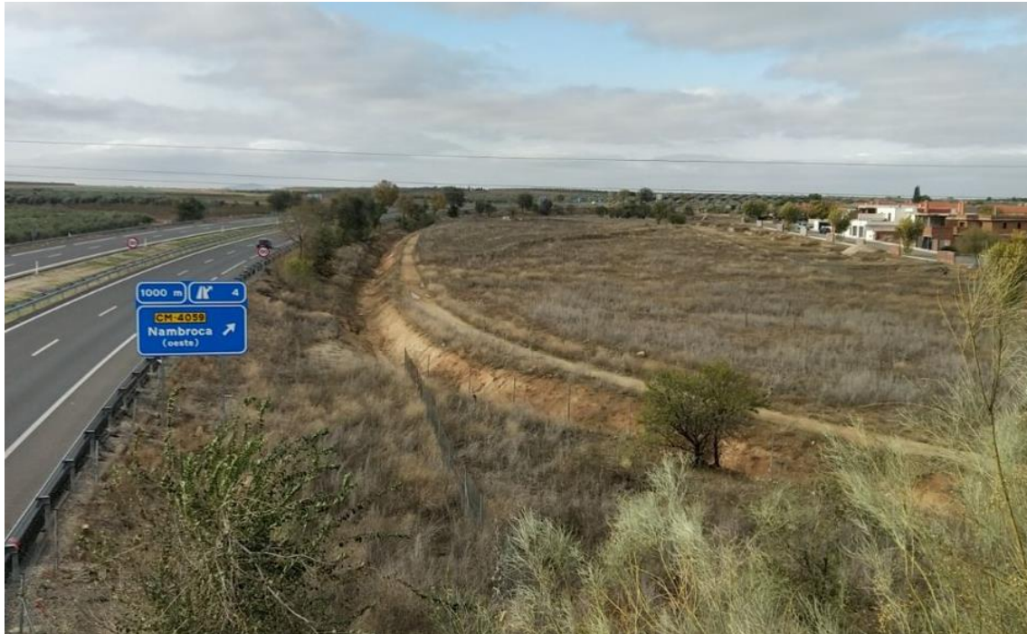
Figure 37: The artificial canal, build to protect the village, was not able to discharge the incoming water and breached at two locations.
