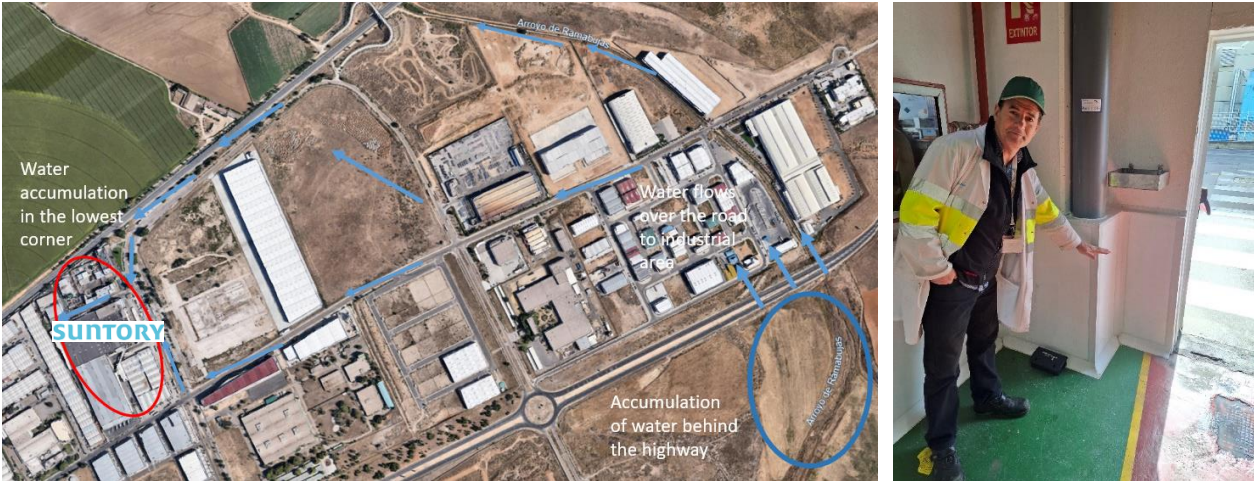
Figure 54: During DANA the water flooded the industrial site and accumulated in the lowest corner at the Suntory factory. Water levels exceeded 50 centimetres in both the factory and the Suntory water treatment plant.
