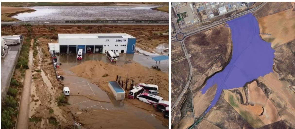
Figure 22: Based on the DEM (Digital Elevation Model) a reconstruction could be made of the lake that emerged during DANA (lake is visible in the left drone image from the day after). More than 900.000 m 3 of water was temporarily stored on area of 28 ha (bottom).
