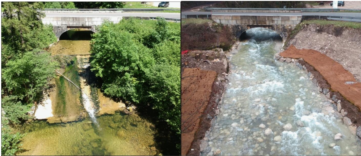
Dalloz dam (France) before and after removal.
