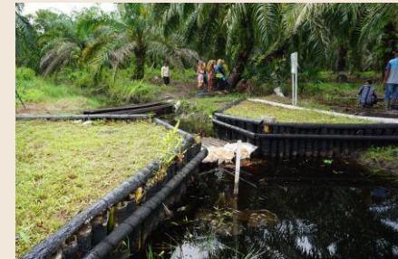
Canal blocking effectively blocked the water in the upstream
